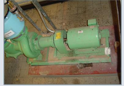
Pump used in wastewater facility that has been secured to a LOCTITE® Grout base
