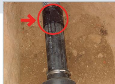
Pipe coupling repaired with LOCTITE® MR Flex 80™ Urethane Repair
