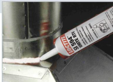
Ductwork being sealed with LOCTITE® SI 594™ Silicone Adhesive Sealant
